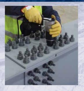
Standard TCB® - used in a wide range of steelwork connections from bridge splice plates to beam-to-column connections, from stadia roof trusses to rail switches & crossings.
